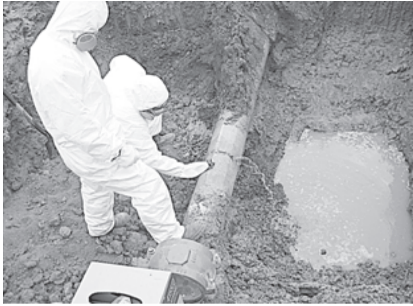
Coober Pedy Water Supply workers repairing damaged boreline wearing asbestos protection
