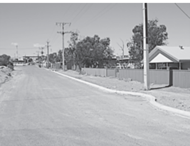
New kerbing in Brewster Street
