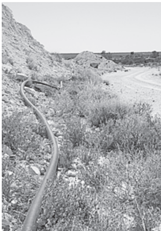
The Mintabie water pipe running into town
